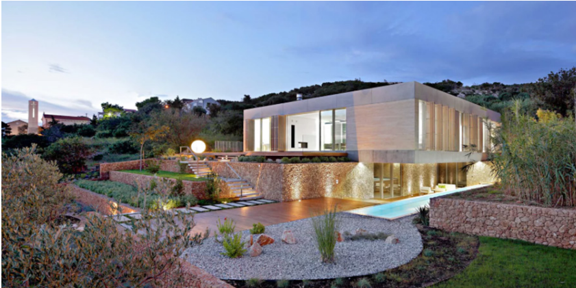
Casa Olivo, Fachada surorientada y surponiente. Fuente: https://architizer.com/projects/olive-house-1/
